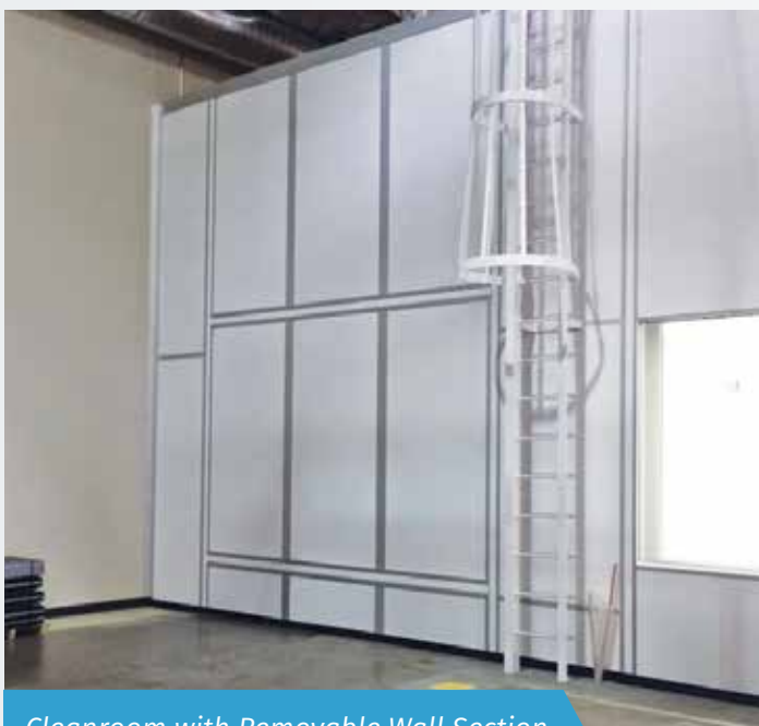
Cleanroom with Removable Wall Section
